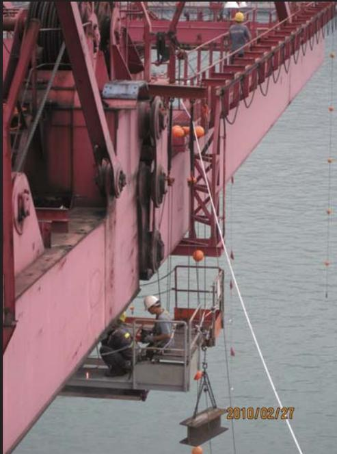
Our Equipment Maintenance Department received a repairing contract earlier this year to replace the boom articulation pin and bush on a goose neck quay crane in Hong Kong. We were provided with the working procedures to follow and expected to complete the work within seven consecutive working days.
